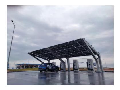
There are 2 fast charging systems for electric vehicles with 200 kW and 2 with 50 kW power within the system.
