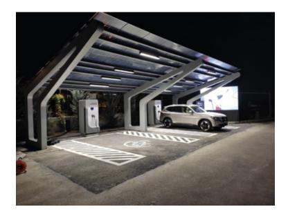
In this project, energy generated from solar energy is stored in battery storage systems completely independent of the power grid, and energy generated from fully renewable energy sources is used to charge electric vehicles.
